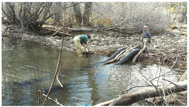
The water is low, and will not flow thru the pipes until water levels rise this winter, to keep pond levels safe for beavers while not flooding trails. By the time we finished, the leveler pipes are hidden with sticks and logs. The cage will be underwater when levels come up, and hide now with a few thinner willow branches on top.
