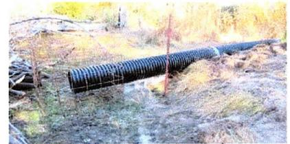
The Conservancy crew dug out the old pipe and inlet cage, and installed and staked new pipe sections (above) to extend past all beaver dams (beavers kept building dams further down the creek). We set the pipe height to keep the pond level safely below the road, if and when beavers return to the site. (The beavers moved elsewhere when the creek dried up the past two dry summers.)
